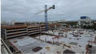
Construction of Park 6 (a seven-level parking structure at MIA) which began on January 4, 2024, continues to progress. This parking garage will include 2,240 parking spaces, two vehicular/pedestrian connections per level to the Flamingo Garage, electrical communication rooms, passenger elevators, 34 oversized vehicle ADA parking spaces and 50 electric vehicle charging stations, including the infrastructure for future additional stations. The target substantial completion date is January 2026.
